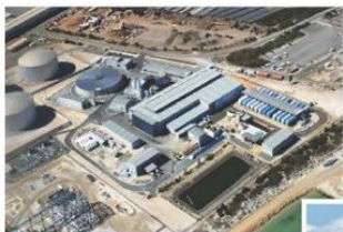
Perth Seawater Desalination Plant 2008
