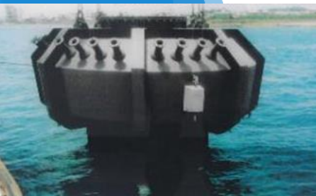
Discharge tower for concentrated sea water
