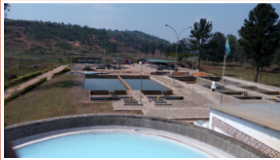
Photo 1: Water treatment plant.
