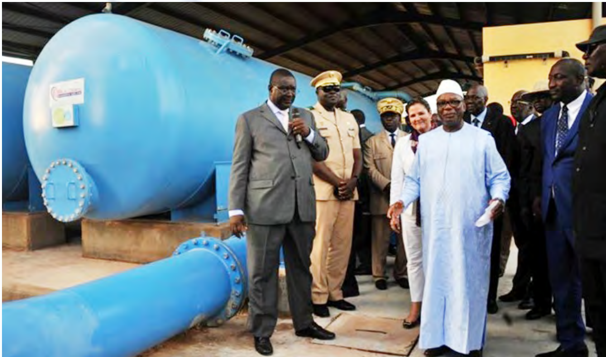
H.E. Ibrahim Boubacar KÉÏTA, Head of state of Mali, visiting the urban wastewater treatment plant
